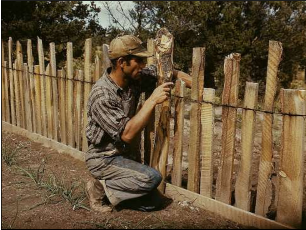
Here, a resident of Pie Town builds a fence with cheap slabs cut with a circular saw and strung together with wire.
