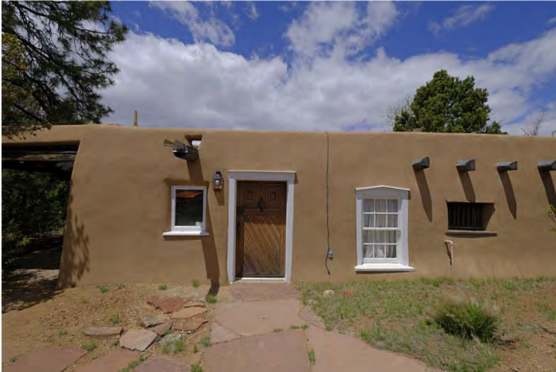
Photo 5. East façade, kitchen entrance, photographer facing west.
