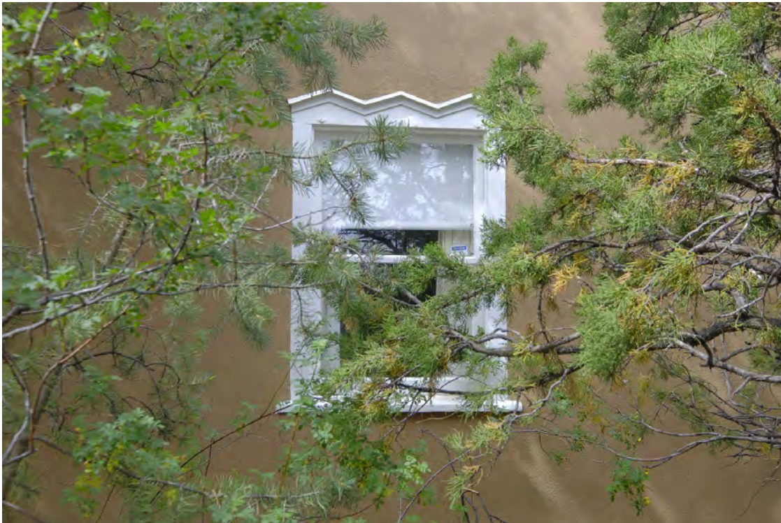
Photo 6. West façade, Territorial Revival-style window, photographer facing east.
