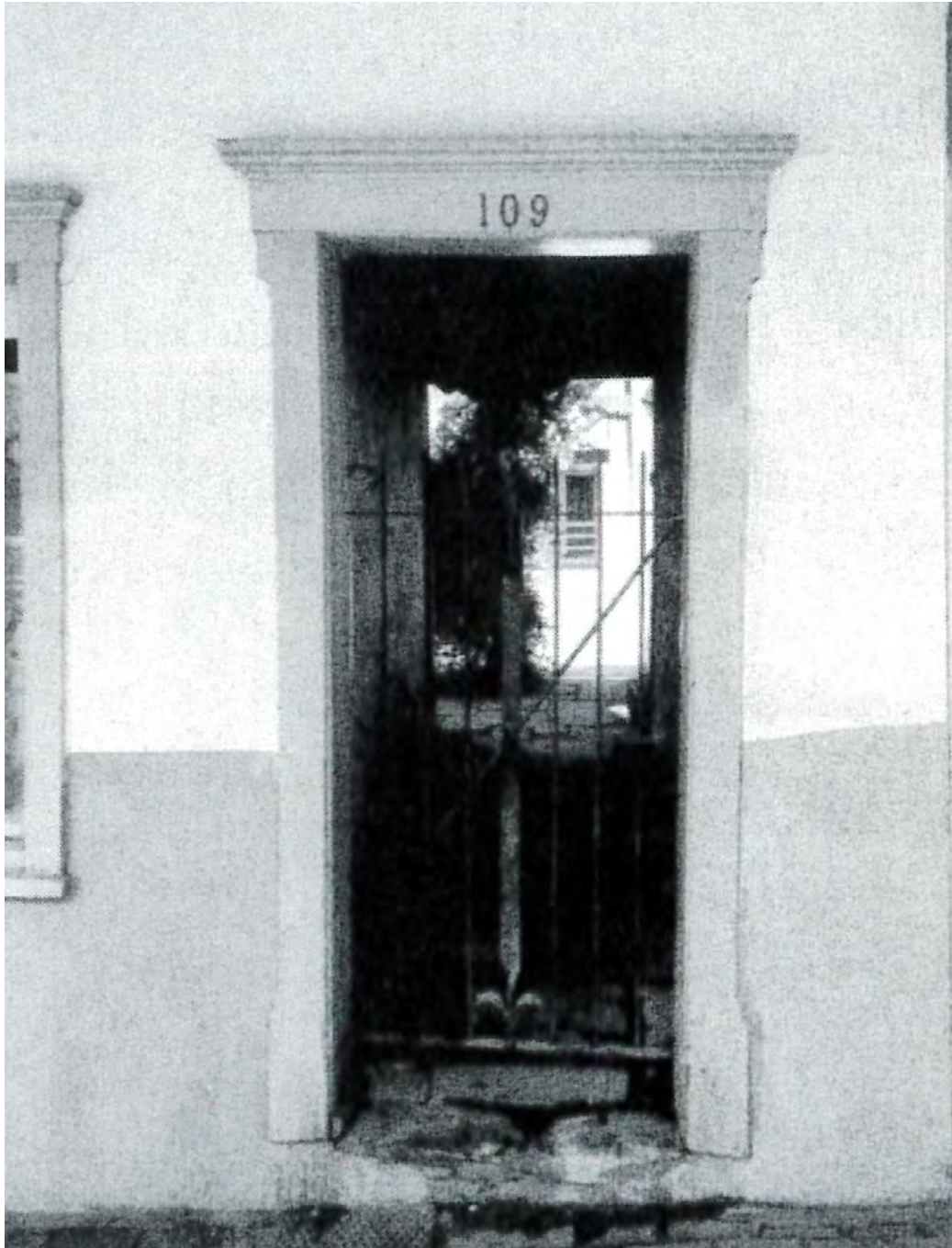
Figure 7. 109 East Palace Avenue, Santa Fe, where McKibbin administered transportation, housing, and communications for newly arrived scientists on their way to Los Alamos.
