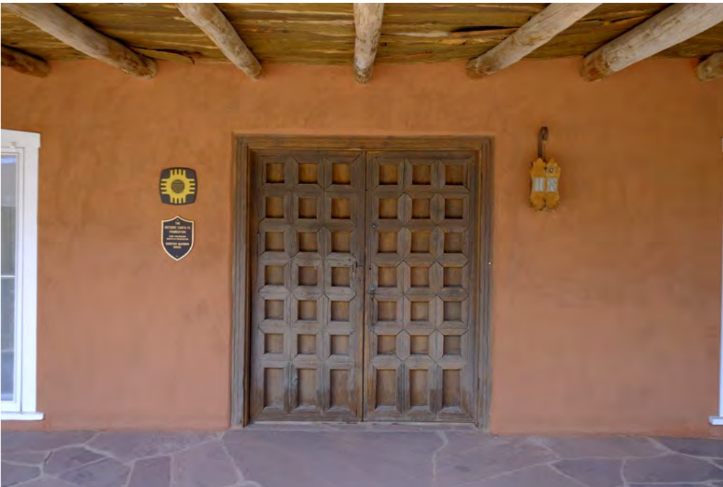
Photo 4. Main portal, paneled door, photographer facing south.
