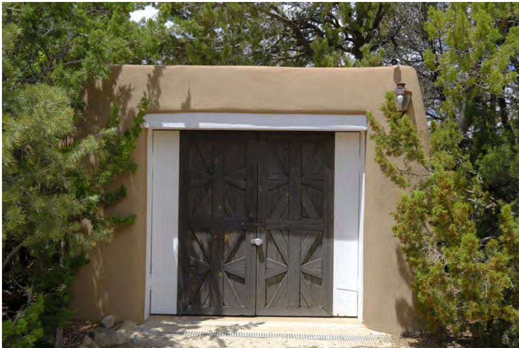
Photo 8. Attached garage with paneled door, photographer facing west.
