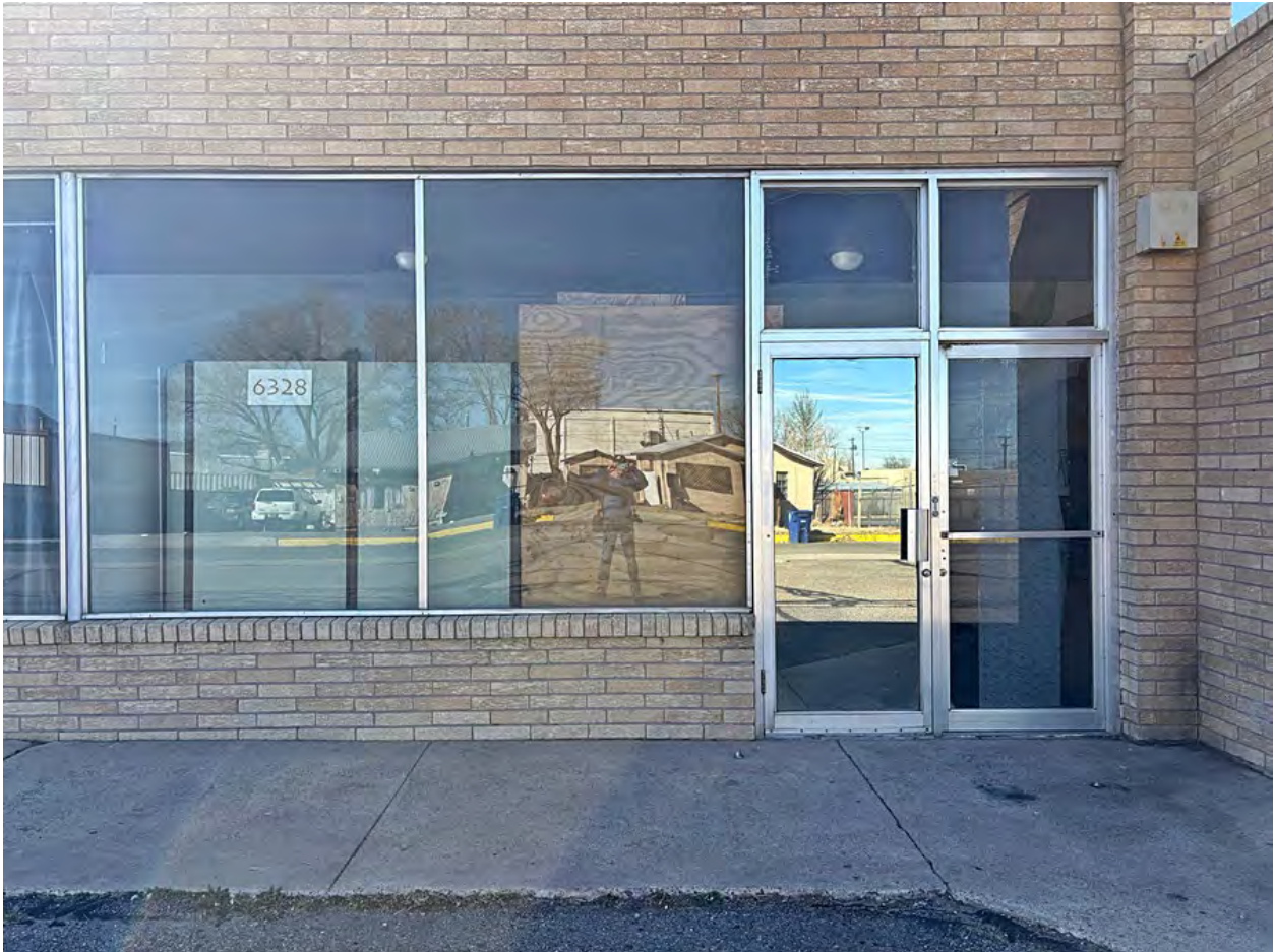
4 of 11. North elevation, Suite 6328, entry detail. Camera facing south. March 1, 2026.
