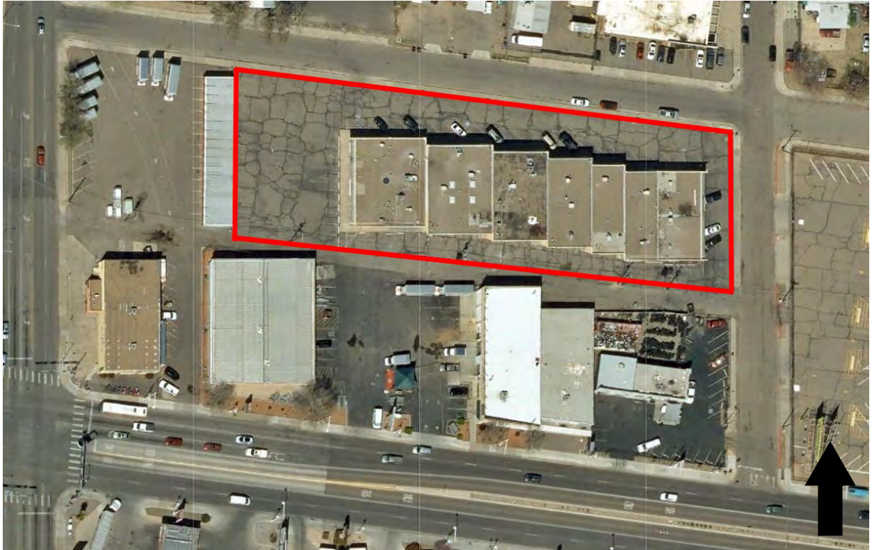
Figure 2: Satellite image of Cal-Linn Building (MITS and Microsoft Headquarters). Boundary highlighted in red. Approximate scale: one inch = 115 feet.
