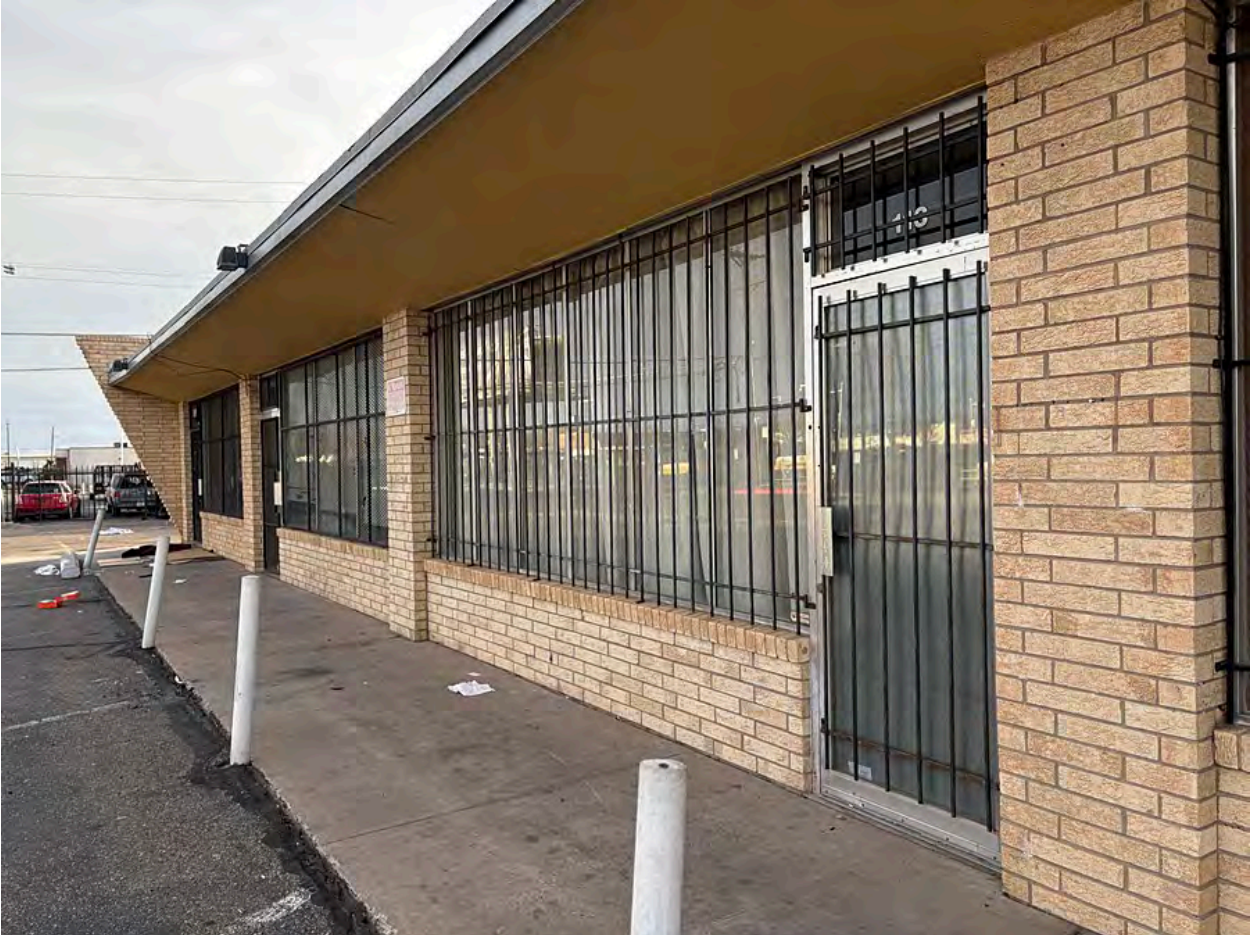
5 of 11. East elevation. Camera facing southwest. February 7, 2026.
