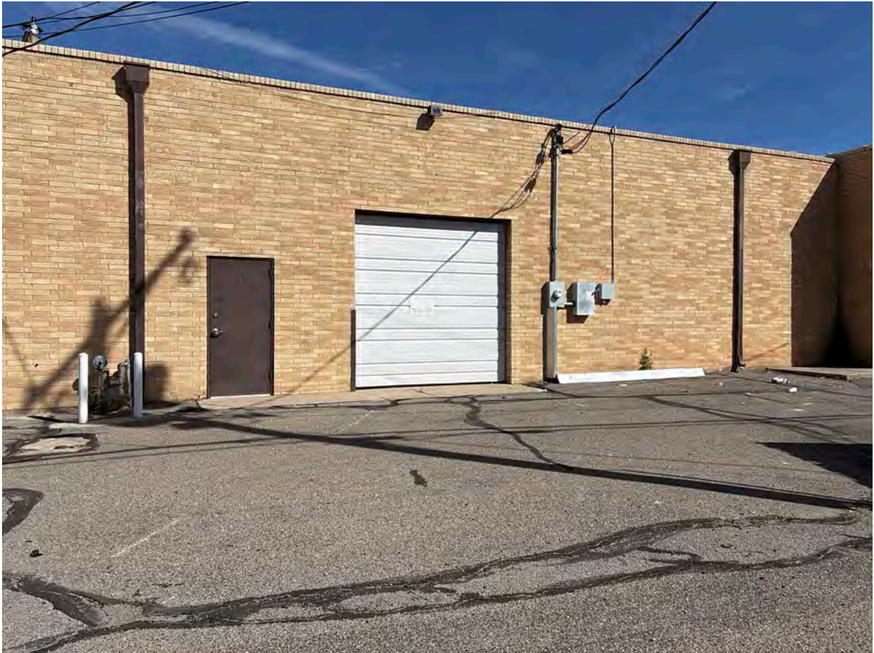
8 of 11. South elevation, loading door to Suite 6328. Camera facing north. March 9, 2026.
