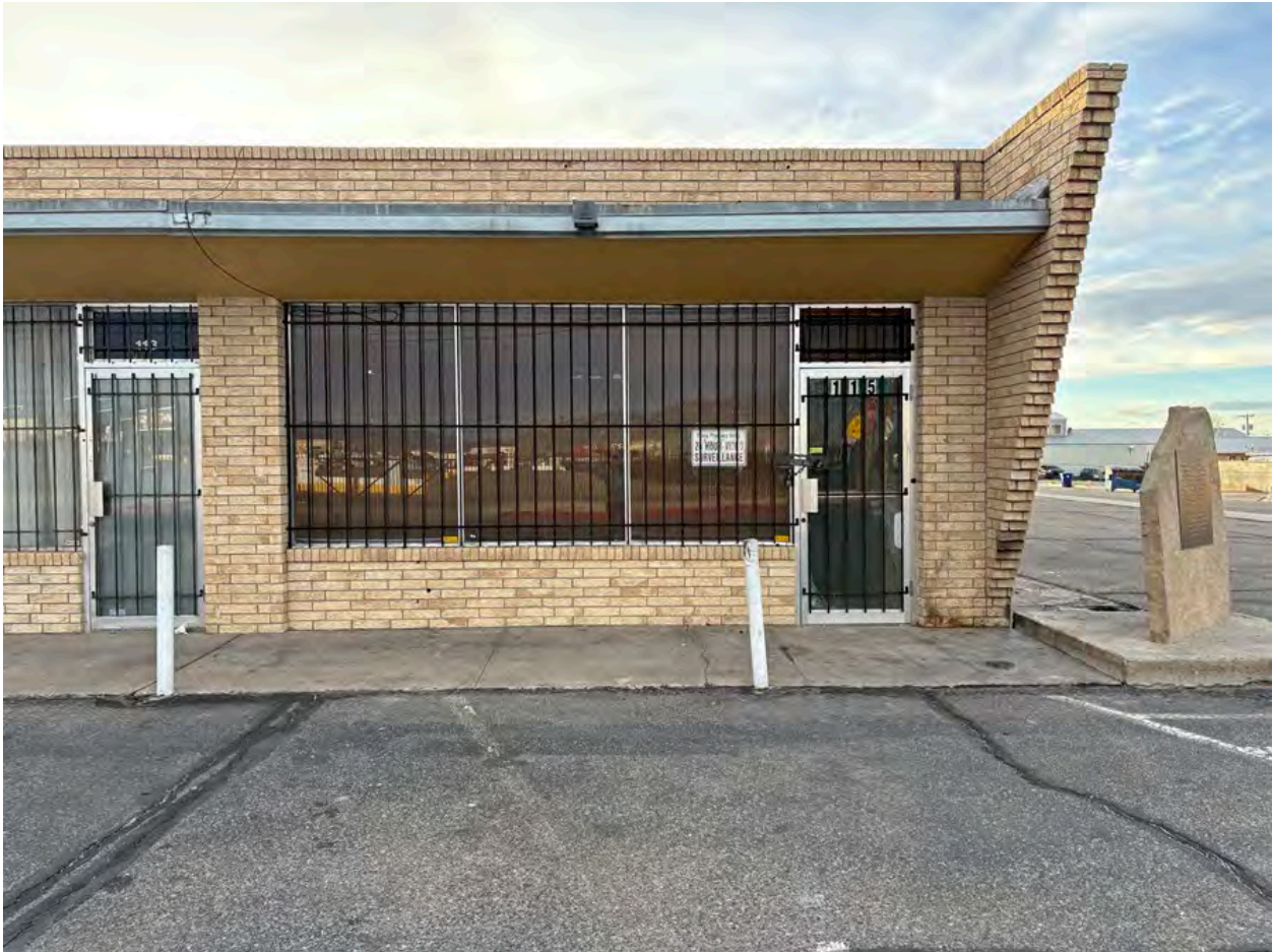
6 of 11. East elevation, Suite 115. Camera facing west. February 7, 2026.
