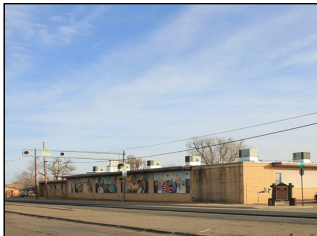
The Lincoln-Jackson School in Clovis, New Mexico, was listed in the National Register of Historic Places in 2017
